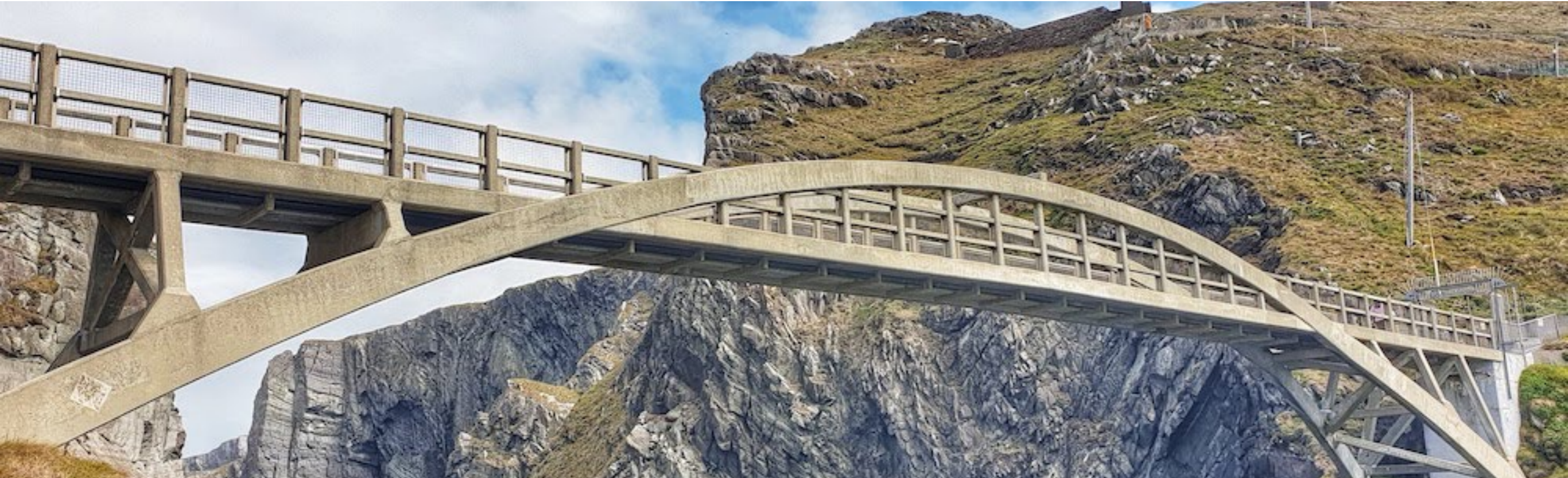
Mizen Head bridge
